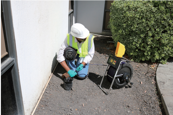
Proper placement and pushing force
